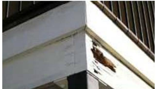
**Check bearers and joists for warping or cracking.**
