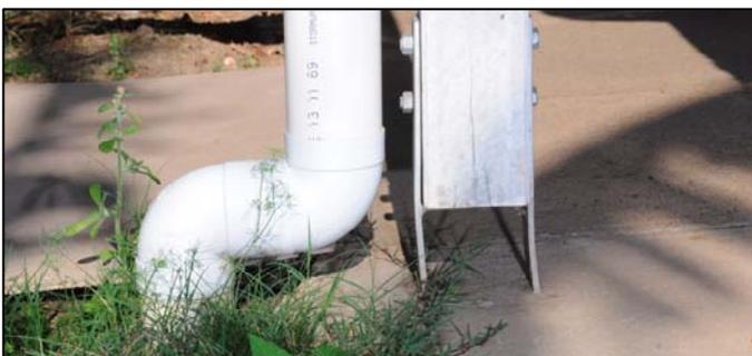
Inspect post brackets for bending or stressing.
